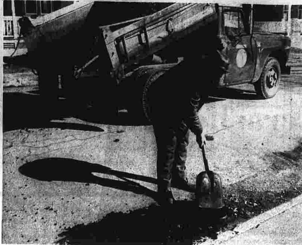
Filling the potholes
